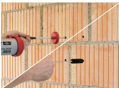
**Assembly with threaded rod and adhesive mortar**
