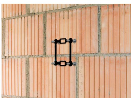
Position the threaded rods and align them exactly by inserting the respective support.
