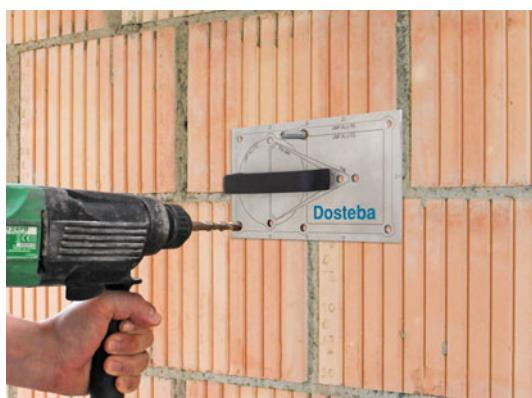
With the drilling gauge for UMP® / TRA-WIK® / TWL®, insert a threaded rod into the corresponding hole.
